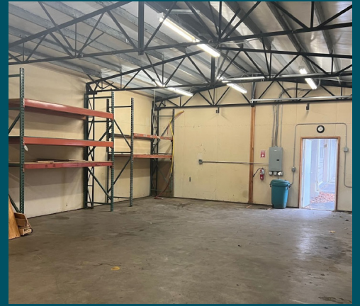
Warehouse with 3 Phase power
