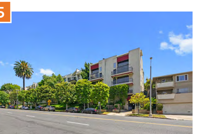
222 Arch St | Laguna Beach, CA 92651
