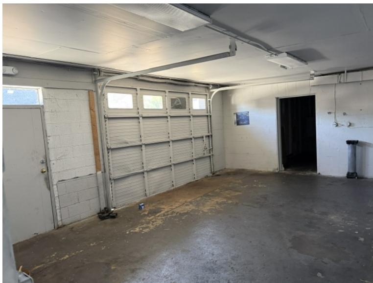
930 S Chapman drive-in bay — roll-up door, 8' clear height, concrete floor. Adjoins the finished office and waiting area.
