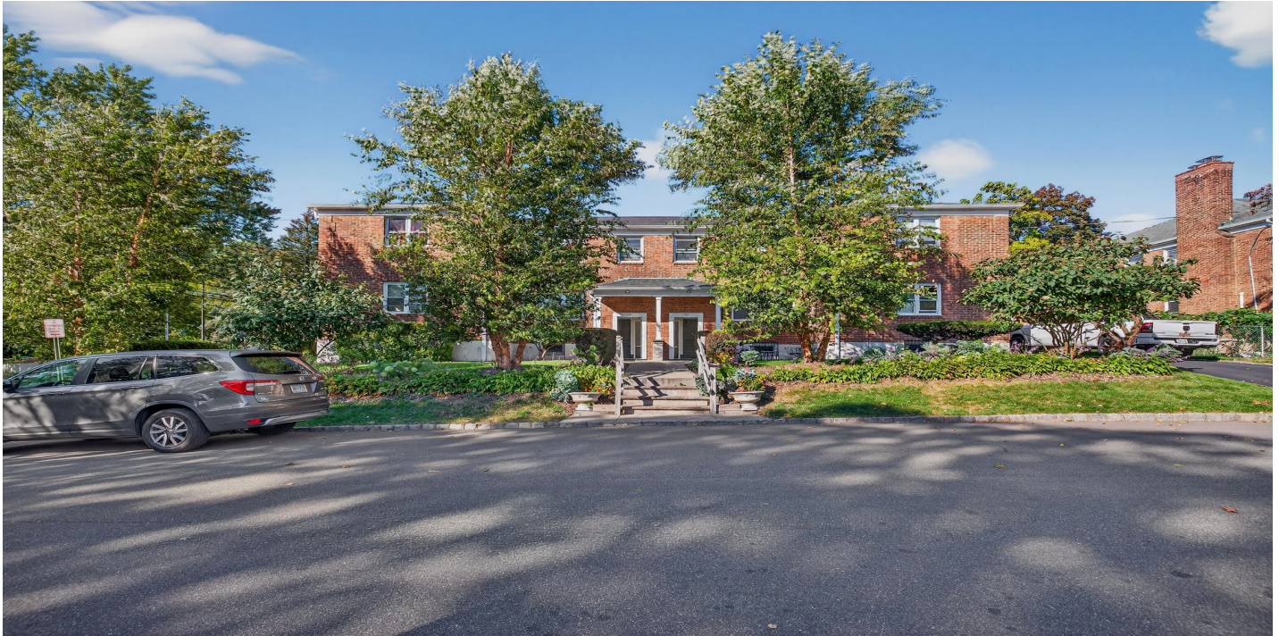
STREET VIEW — Linden Street (26 & 28 Linden St)
