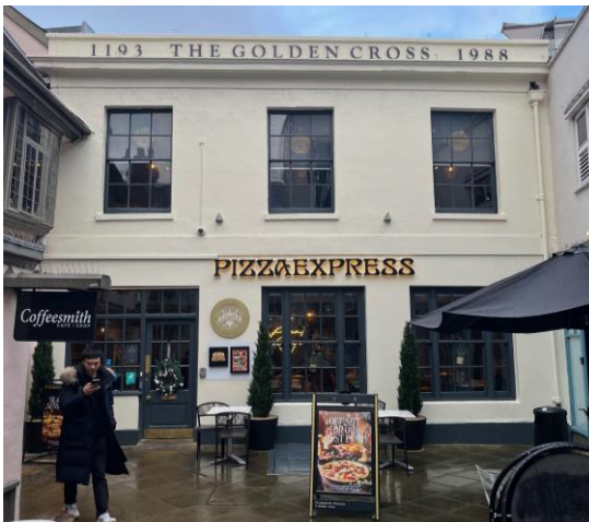
Refurbished Pizza Express Restaurant
