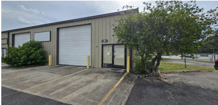
Suite D entrance and grade-level roll-up door
