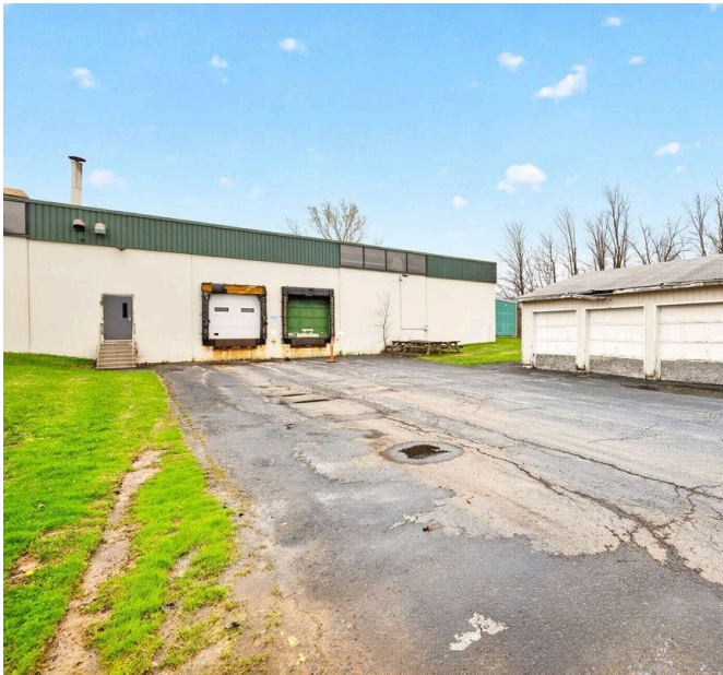
Dock-High Loading Doors & Yard Area
