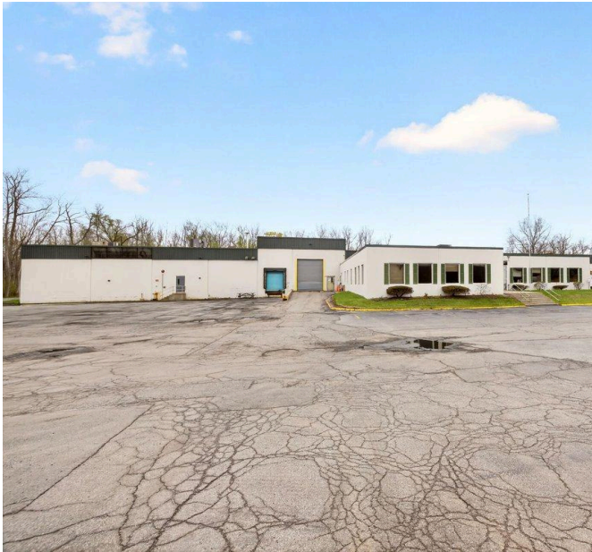
Main Entrance — Office/Reception Area
