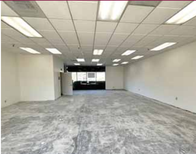
3093 McKee Road - Interior
