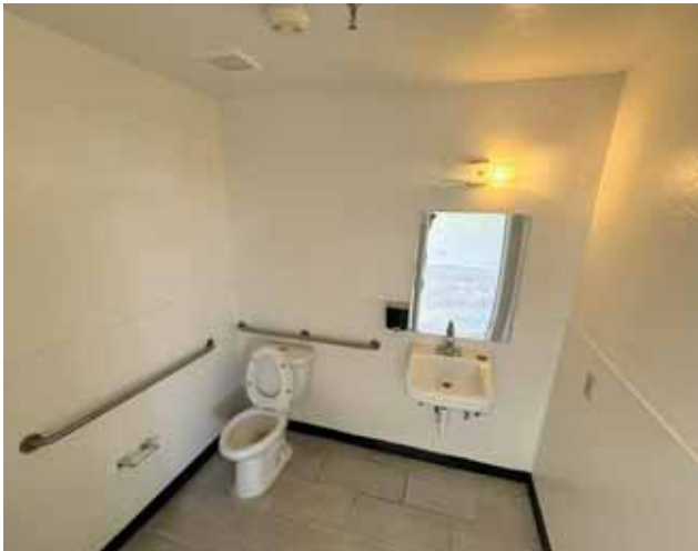
3093 McKee Road - ADA Restroom
