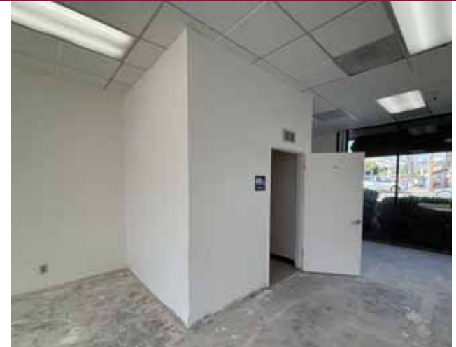
3093 McKee Road - Interior
