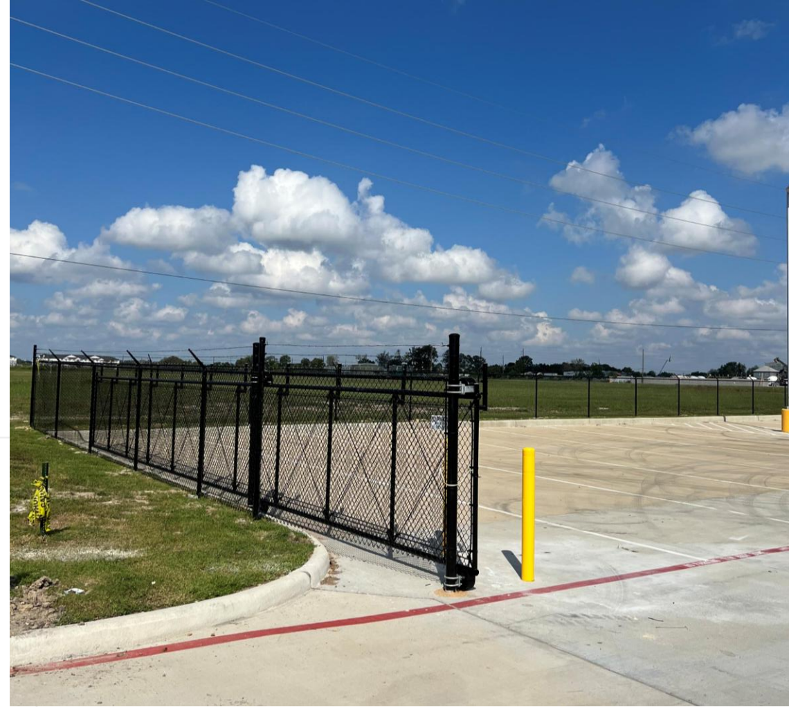
Fully Fenced Backyard with Electric Access Gate
