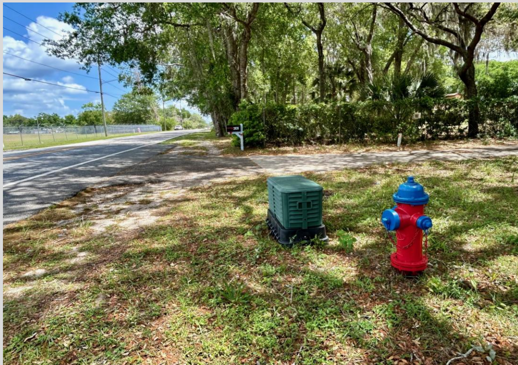
View ROW showing water hydrant and Cable
