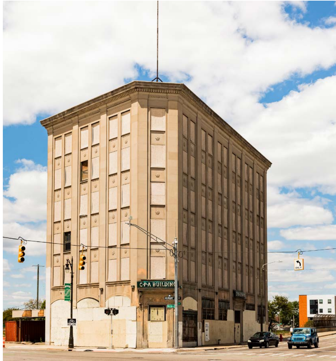
2411 14th Street (CPA Building)
