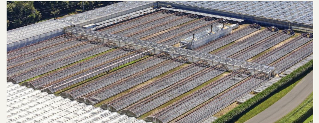
02 Glass roof and bay detail
