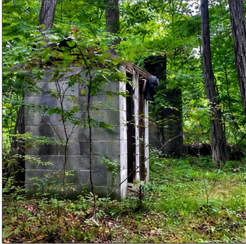
A - 3 Outbound structure (foreground) and portion of store wall (background).
