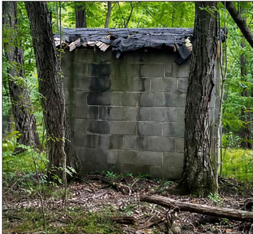
A - 4 Rear view of outbound structure.
