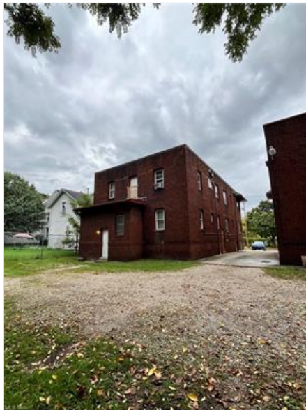
Back of Structure
