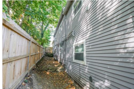
Back of Structure
