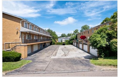
Side of Structure
