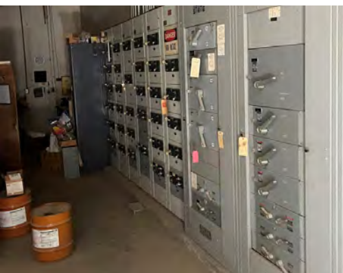
Washington Street E - Mechanical Warehouse
