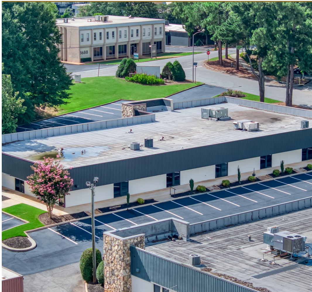
FULL BUILDING / RESTRIPE PARKING FIELD
