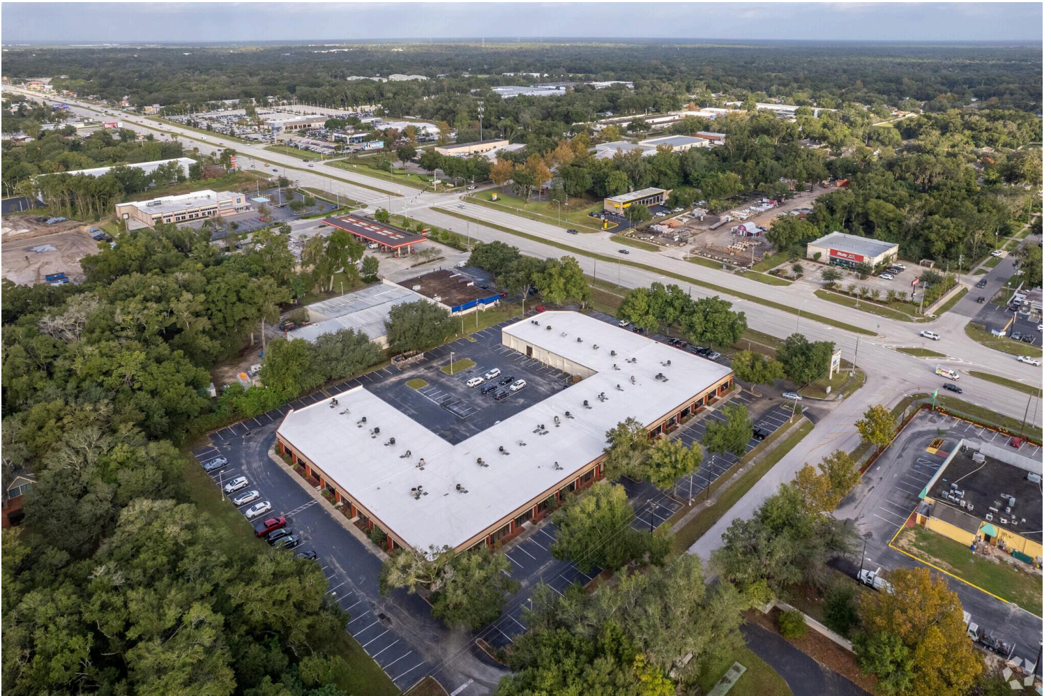
The Wekiva Executive Center has high visibility, facing onto Semoran Boulevard (SR-436), a major thoroughfare in the Orlando area, in the heart of a region that is exploding with growth.
