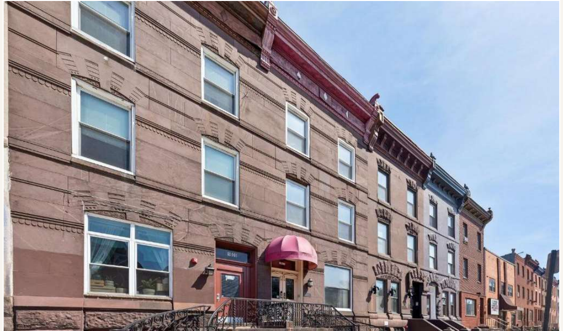
BROAD STREET FRONTAGE
