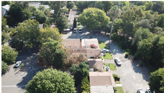
102 Elliott Street, seven residences on 21,250 square feet
