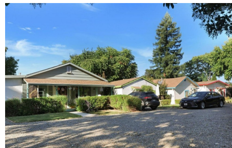
Covered porch cottage, 102 Elliott
