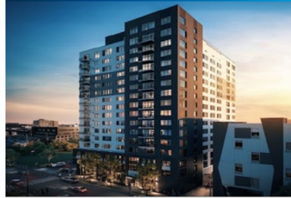
2 3595 WYNKOOP ST Denver, Colorado
