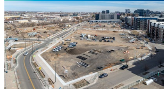
6 2650 ARKINS COURT Denver, Colorado
