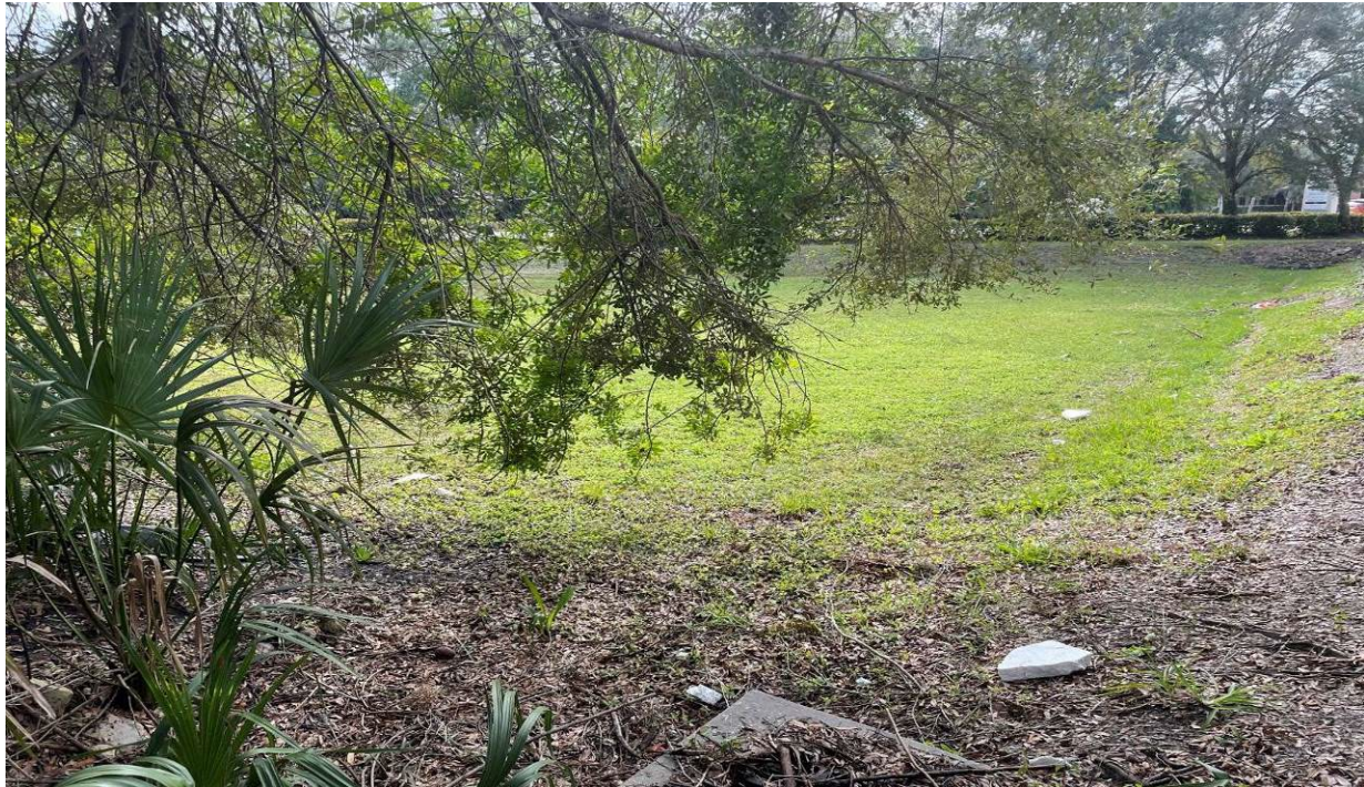
Photo Number: 1 Description: View facing south from the southeast culvert and ditch toward the stormwater basin. Photo date: 1/20/2022 Direction: S
