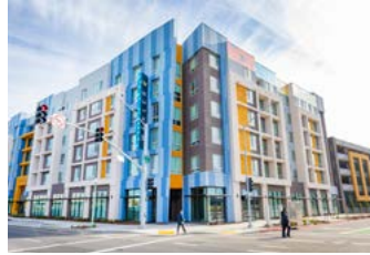
THE WEXLER STUDENT HOUSING Built in 2022, The Wexler is off-campus student housing with 200 apartments and 800 beds.
