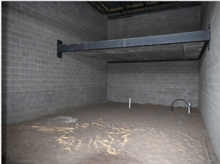
Standard Unit with Dirt Floor and Rough-ins
