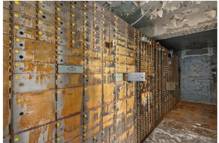
EXPANSIVE VAULT ROOM
