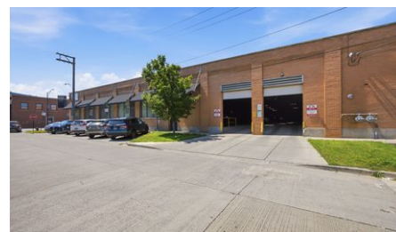
REAR ACCESS · OVERHEAD DOOR
