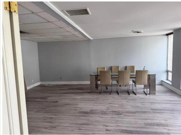
Photo 4. View of a portion of the office space within the subject property, finished with laminate flooring, drywall walls and ceiling, and acoustic ceiling tiles.
