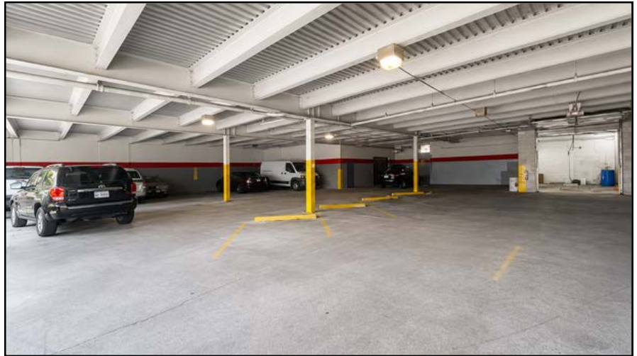
GROUND LEVEL PARKING GARAGE
