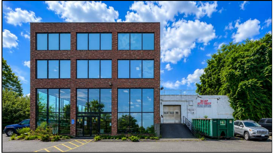
SIDE ENTRANCE TO SHOWROOM & DRIVE-IN DOOR
