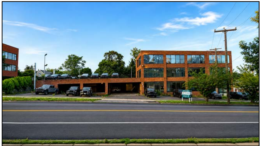
EXCELLENT EXPOSURE WITH 235 FEET OF FRONTAGE ON ROUTE 58
