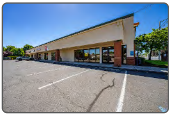
Front Facade & Entry
