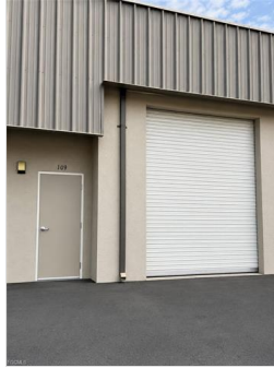
Commercial exterior featuring a large roll-up door, stucco finish, and a corrugated metal upper facade
