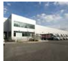
Dunkin' Northeast Distribution Center Bellingham, MA 410,000 SF Completed in 2005
