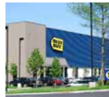
Best Buy Distribution Center Bellingham, MA 239,000 SF Completed in 2009
