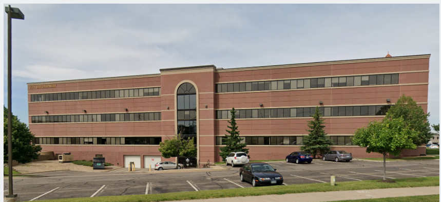
Back of Building
