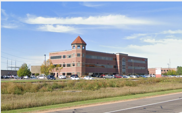
Side/Front of Building
