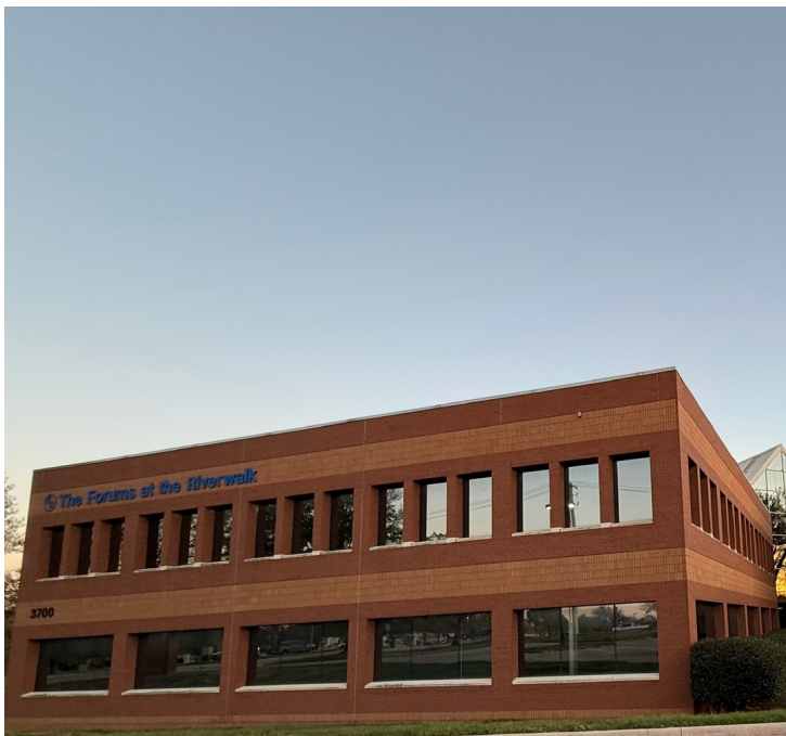
Side Building View
