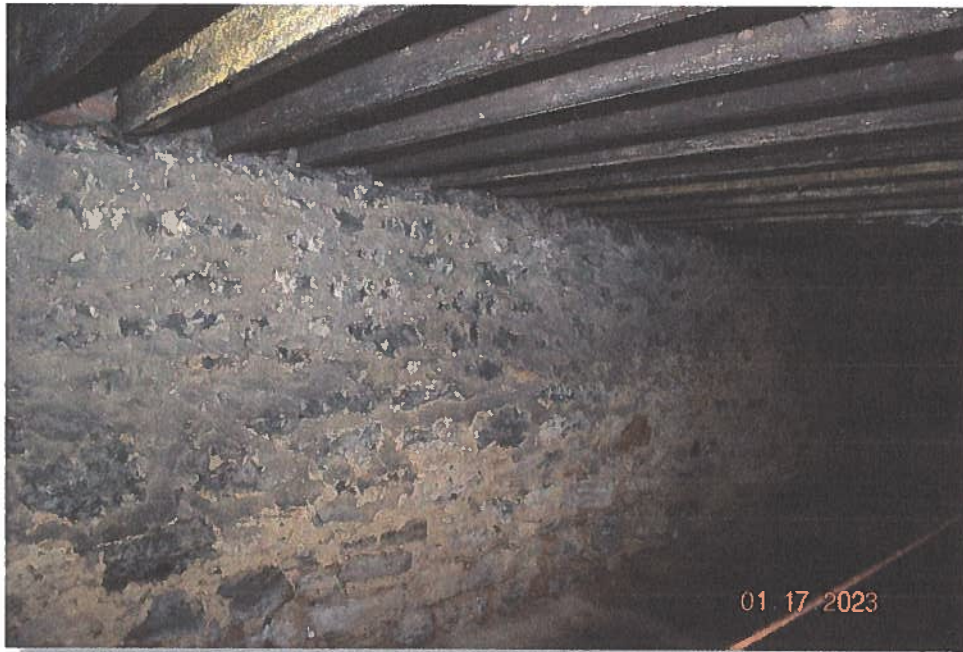
Pic. 15: Typical view of the foundation (interior wall) of unit #1085
