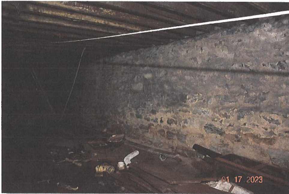
Pic. 16: Typical view of the foundation (interior wall) of unit #1085
