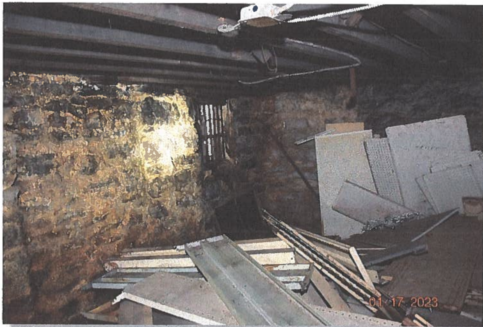
Pic. 4: Typical view of the foundation (inexterior wall) of unit #1083
