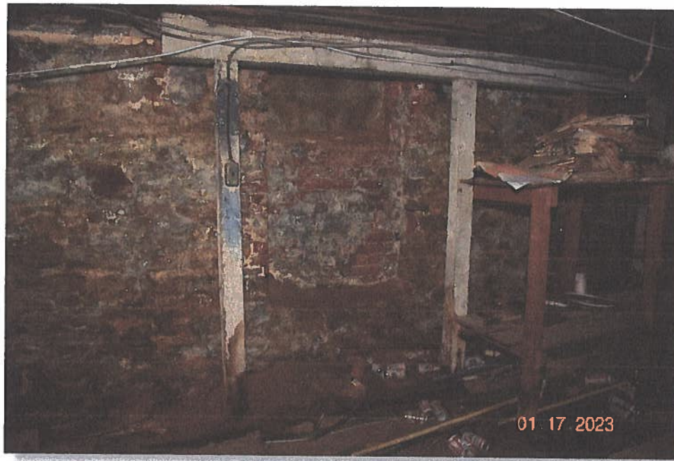
Pic. 17: View of the first-floor level joist framing exterior support @ unit #1081
