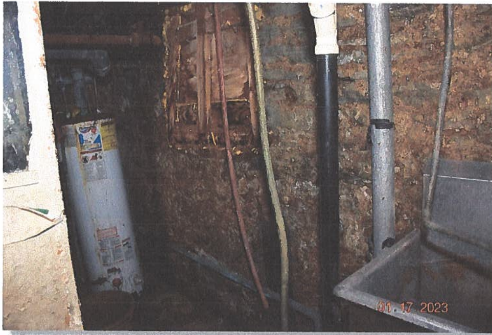
Pic. 1: Typical view of the foundation (exterior wall) of unit #1081
