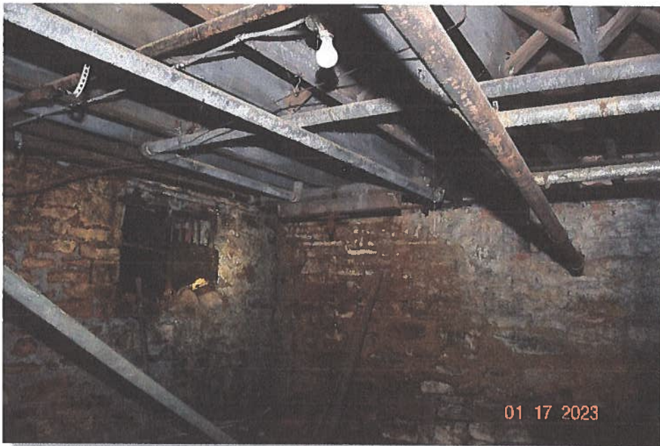
Pic. 10: Typical view of the foundation (interior wall) of unit #1083
