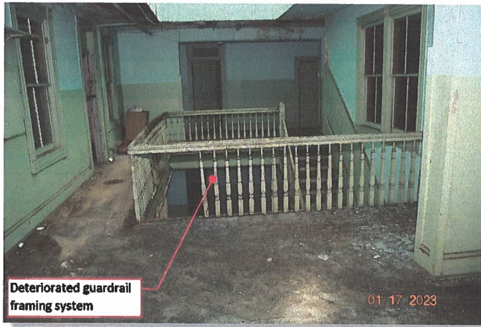
Pic. 31: View of the existing guard rail on the third-floor level
