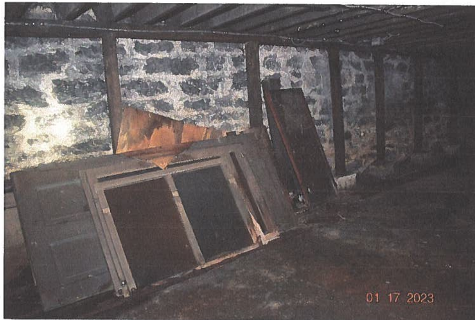
Pic. 14: Typical view of the foundation (exterior wall) of unit #1085
