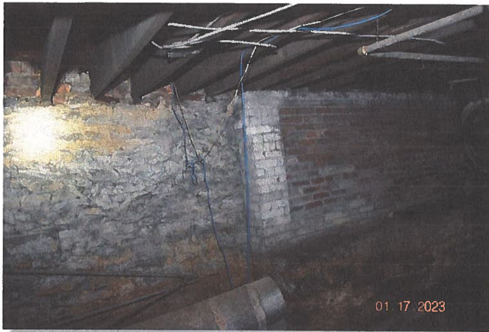
Pic. 9: Typical view of the foundation (interior wall) of unit #1083
