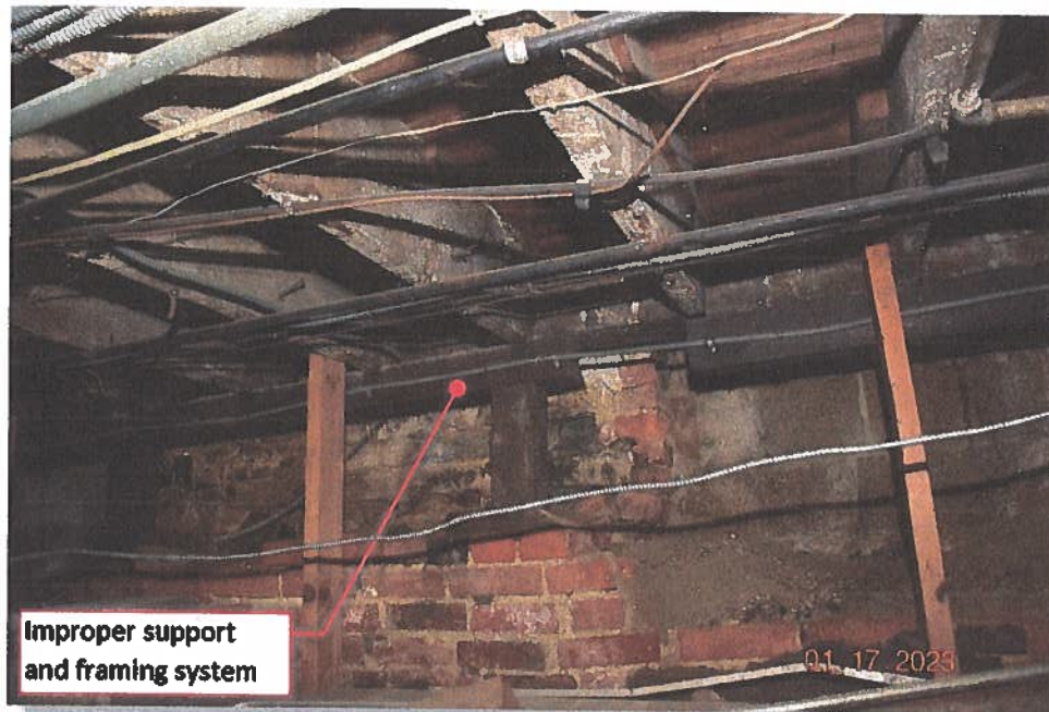
Pic. 20: View of the first-floor level joist framing & support @ unit #1081
