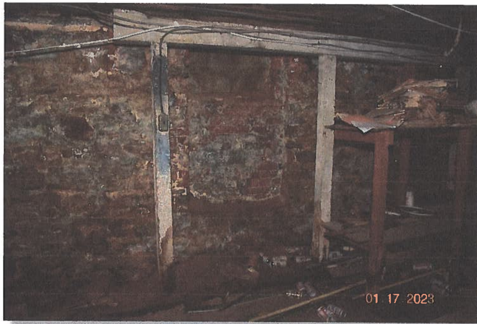
Pic. 3: Typical view of the foundation (exterior wall) of unit #1081
