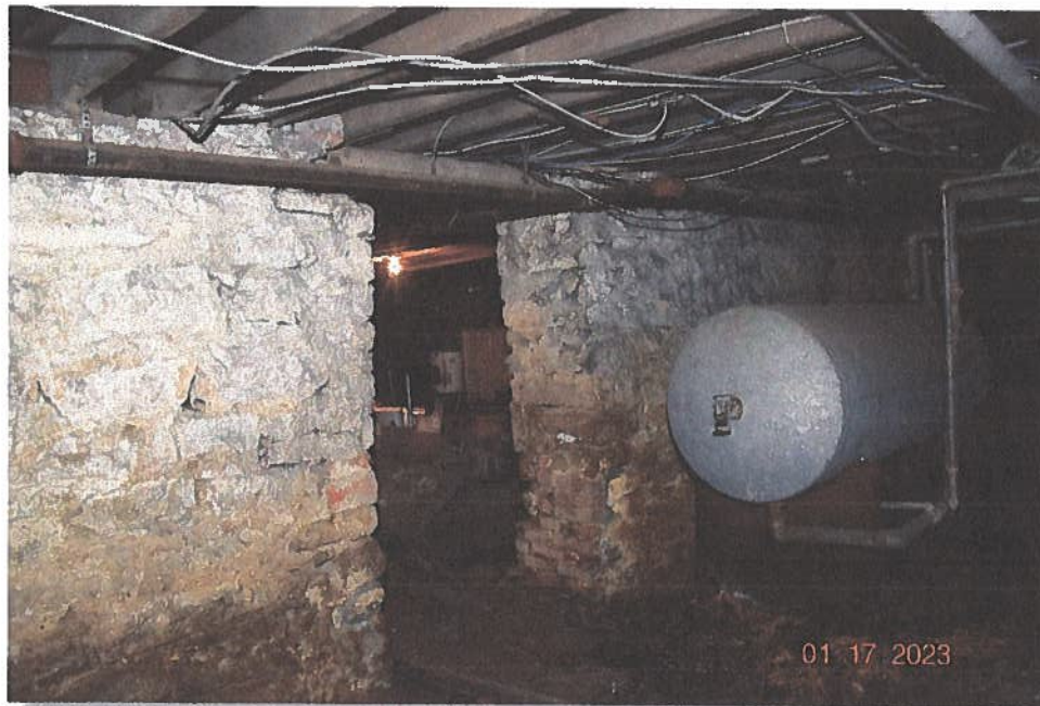
Plc. 8: Typical view of the foundation (interior wall) of unit #1083
