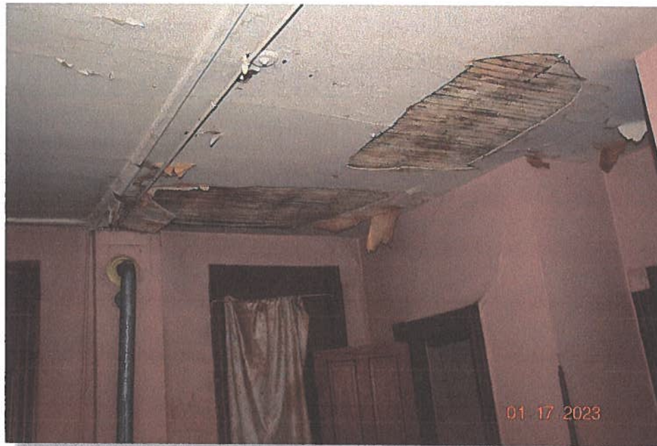
Pic. 28: Typical view of the existing ceiling on the roof level
