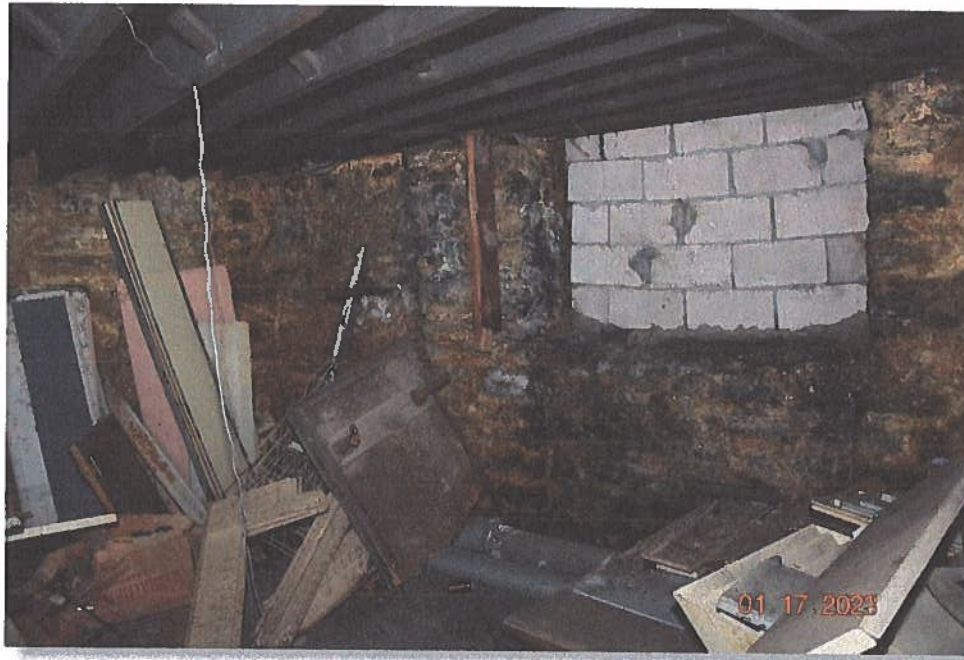
Pic. 5: Typical view of the foundation (exterior wall) of unit #1083
