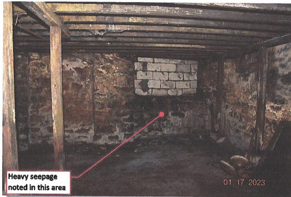
Pic. 13: Typical view of the foundation (exterior wall) of unit #1085
