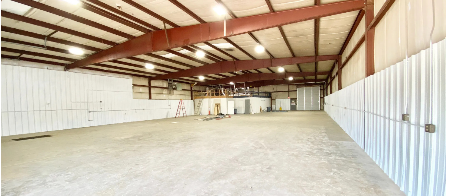
Interior of Warehouse
