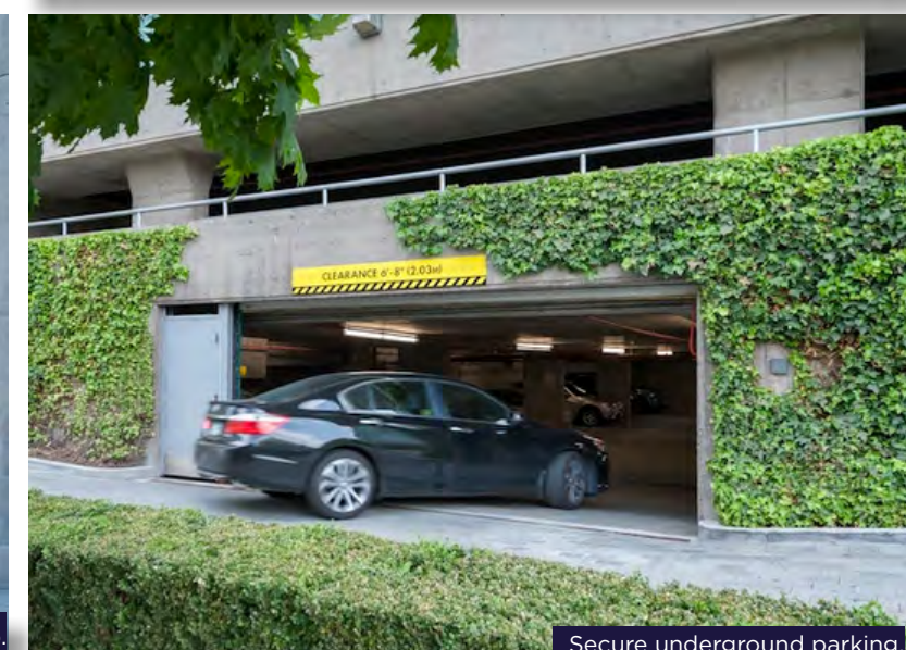
Secure underground parking.
