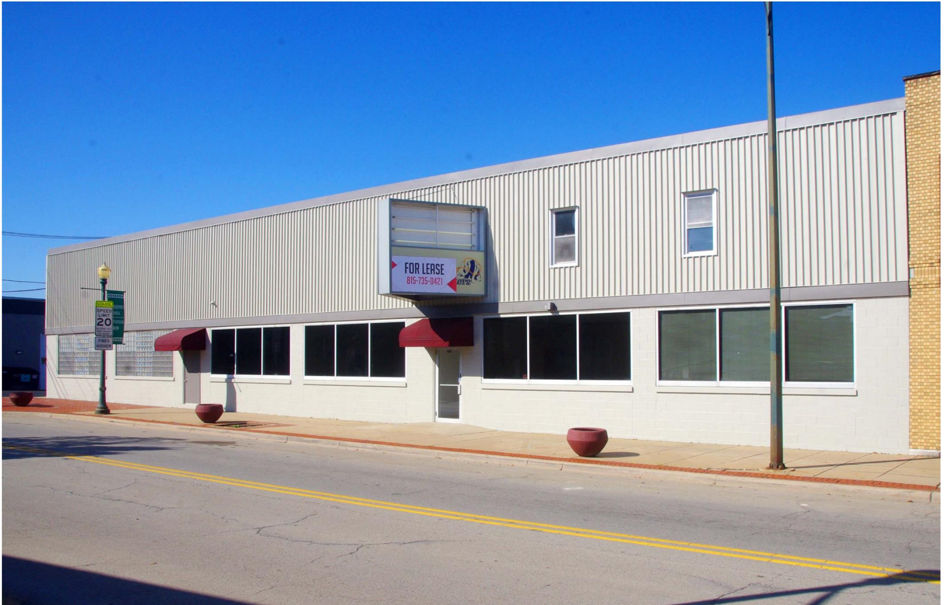
Improved Masonry Clear Span Building – 455 N. Ottawa St. (Rt. 53/66) South West View – Front of Building
