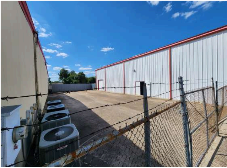
Secure storage between buildings
