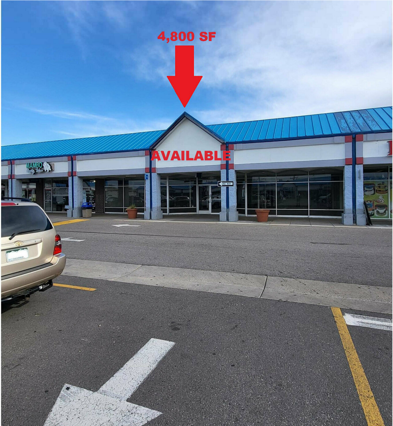
660 Peoria exterior view looking south
