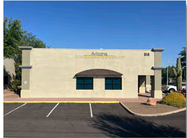
Top: Facing East Bottom: Facing North
