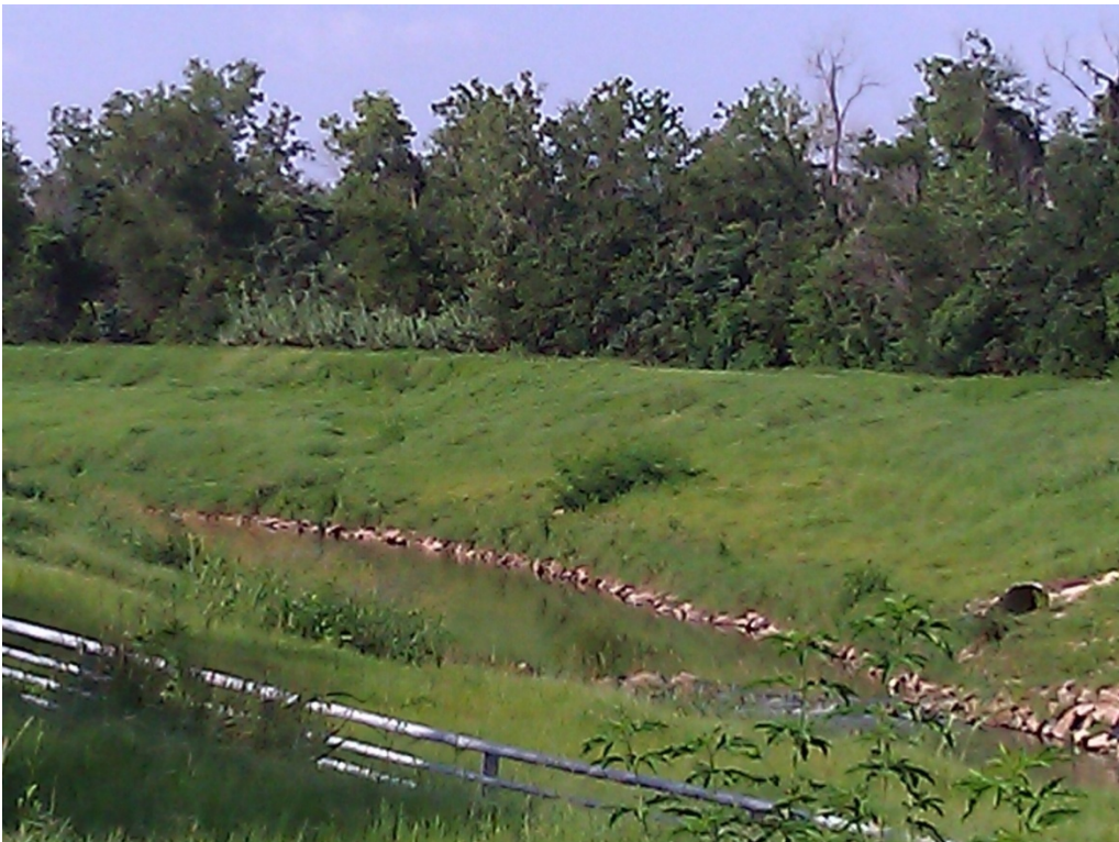
SIDE VIEW LOOKING EAST TOWARDS EXISTING SITE ALONG E100-00-00
