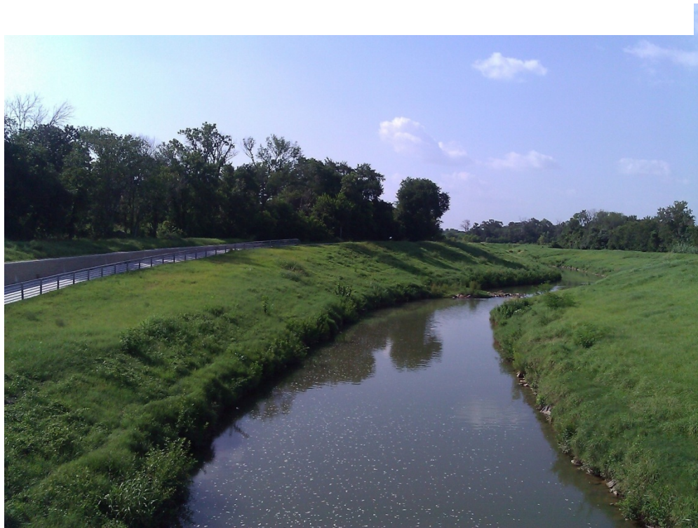
LOOKING DOWNSTREAM E100-00-00 FROM W TIDWELL BRIDGE
