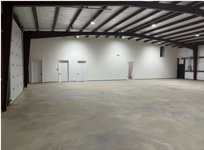
Warehouse interior — open span with LED lighting
