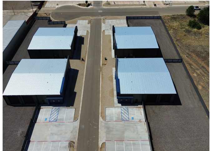
Overhead aerial — all four buildings and parking
