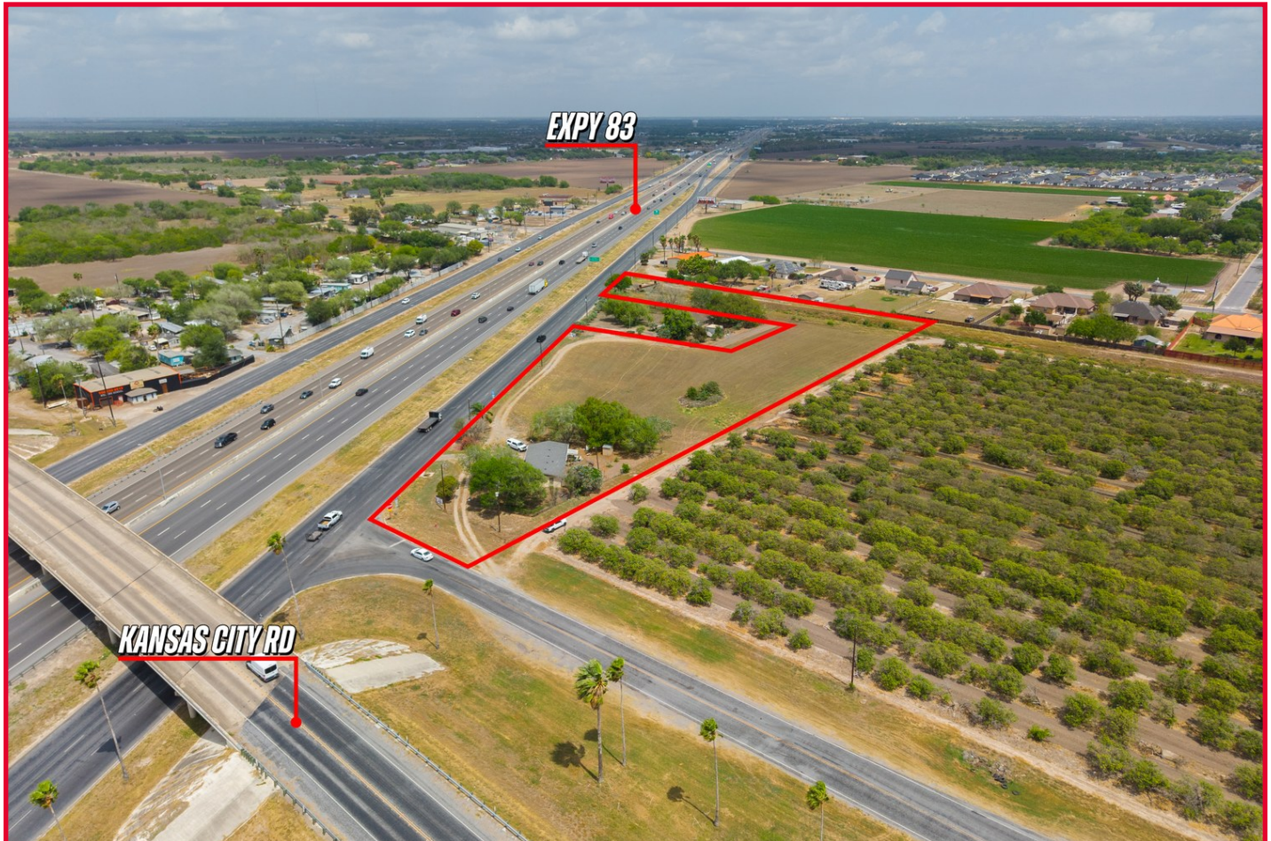
Aerial view with approximate property boundary.
