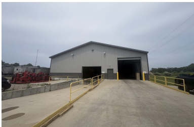
Front Entrance & Loading Docks
