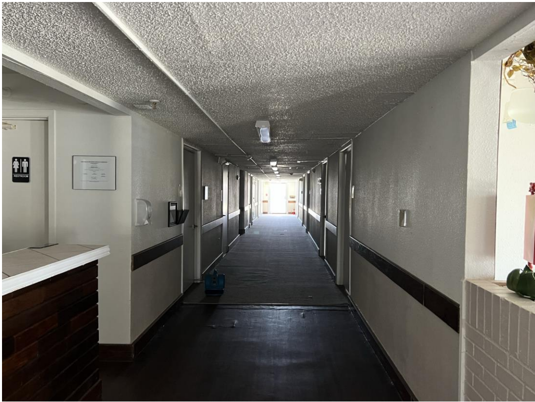
Typical Interior View of the Subject Property
