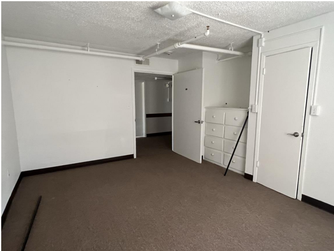
Typical Interior View of the Subject Property
