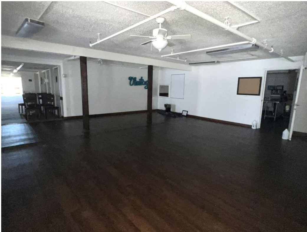
Typical Interior View of the Subject Property
