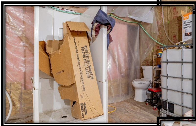
Plumbed For A Bathroom
