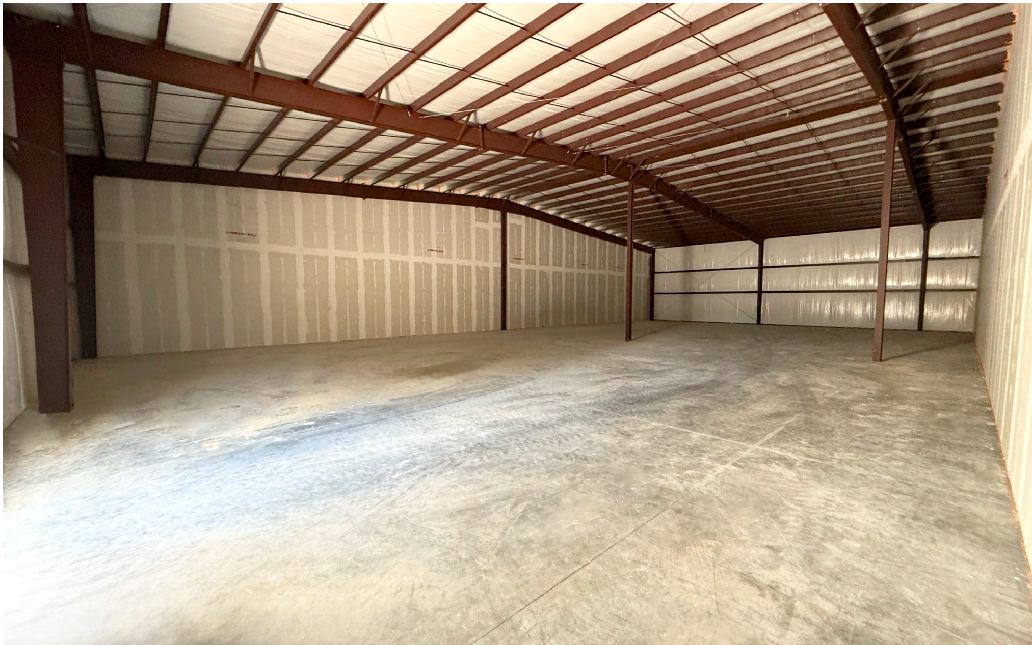
Interior Spaces Construction Progression September 2025
