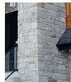
Stone Entrance Piers
