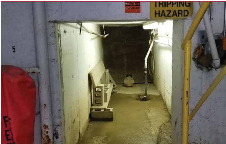
Basement Tunnel to Old Ready-Mix Terminal
