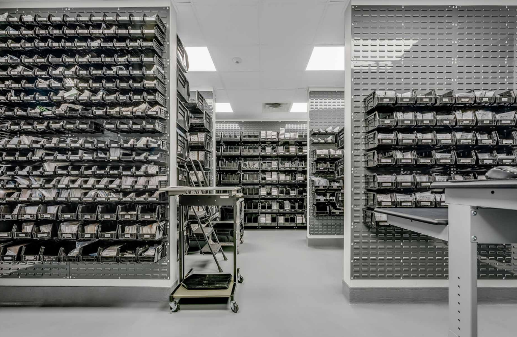
10 Canyon Road - Lower Level.
