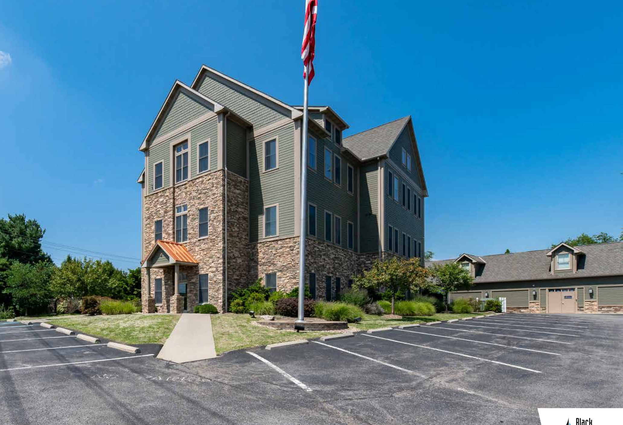
Exterior View, Front of 6 Canyon Road.
