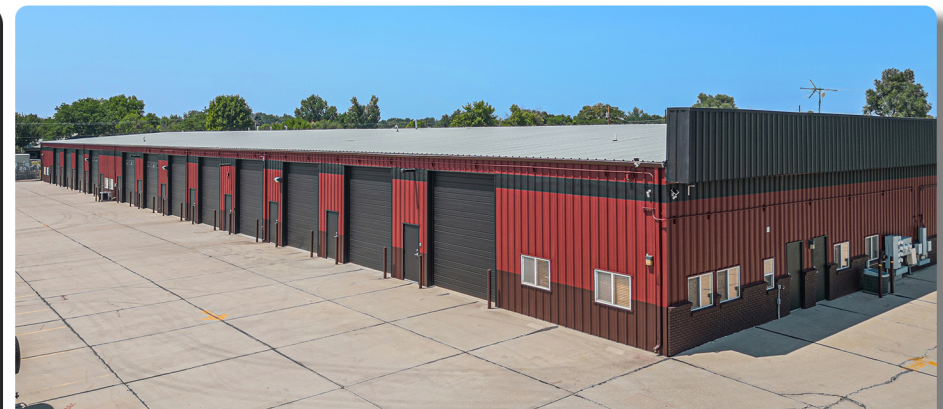
New tenant finishes include bathrooms, offices, monument sign, and exterior paint.
